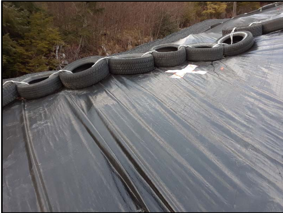
Photo 11: Looking northwest at the treated stockpile and location of TSP-2 after tape repairs to the stockpile cover. Note wrinkles in the cover resulting from tire shifting that occurred during the winter/spring of 2018.
